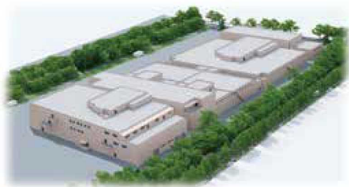
Image of covered purification plant
