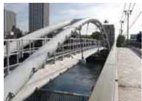
Water Pipe Bridge
